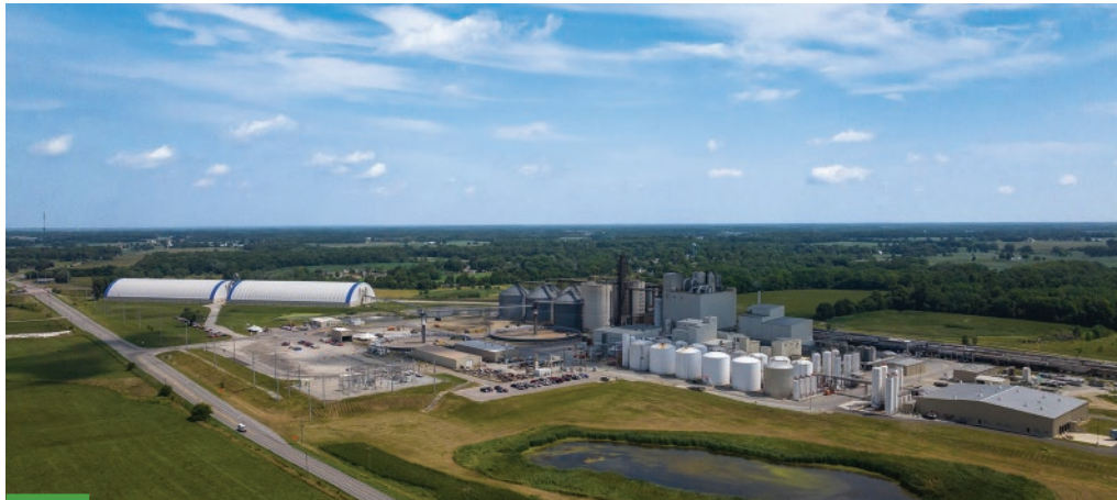
Claypool Plant- US
