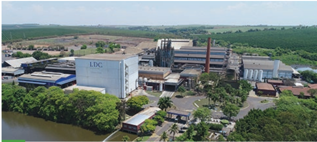
Bebedouro Plant- Brazil
